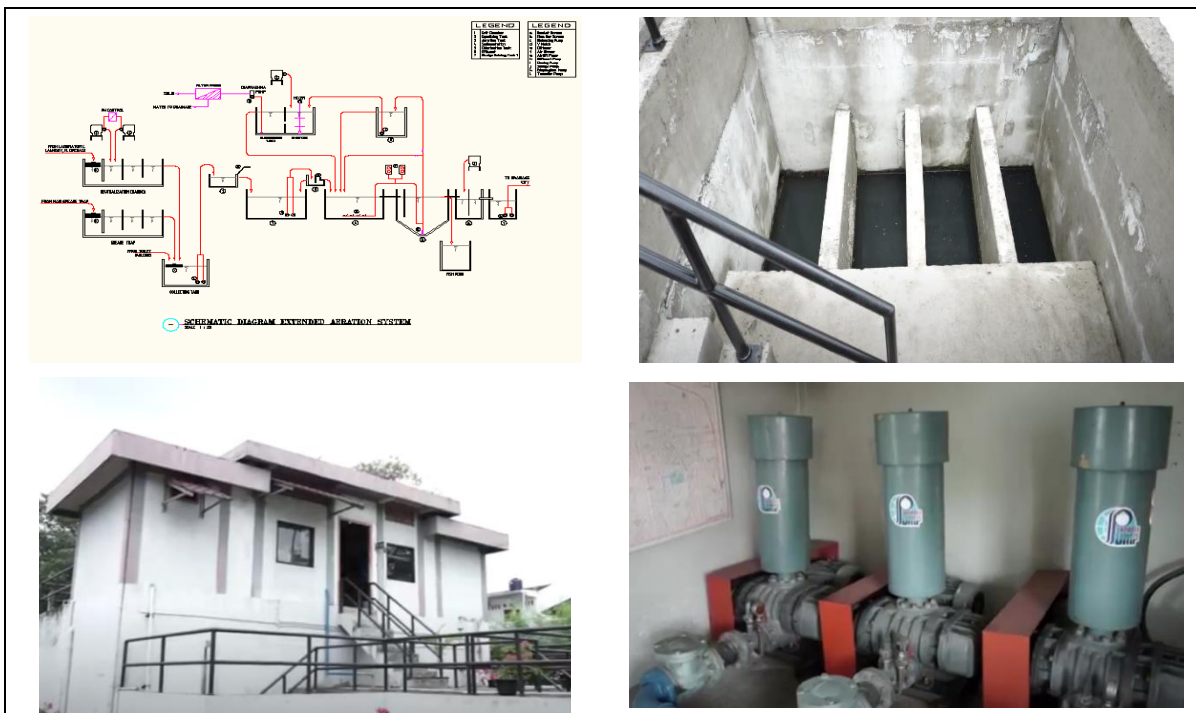
2. Waste Water Treatment Plant at USU Hospital
