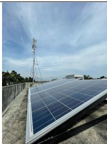
Roof Top Solar Panels in USU Office 21 kWp
