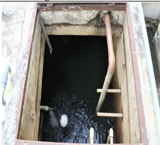
The Use of Water Tanks Equipped with Automatic Float Ball at the Faculty of Public Health, USU
