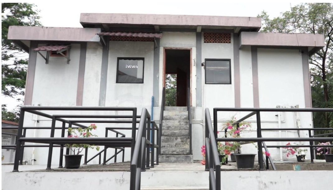
Wastewater Treatment Plant at USU Teaching Hospital
