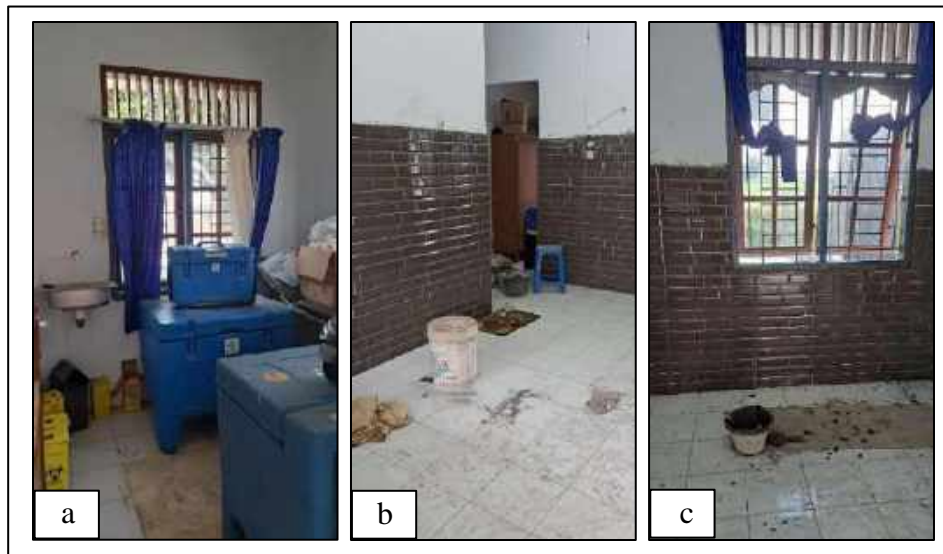
Gambar 4. Renovasi ruang UPT (Unit Pencegahan Terpadu)
