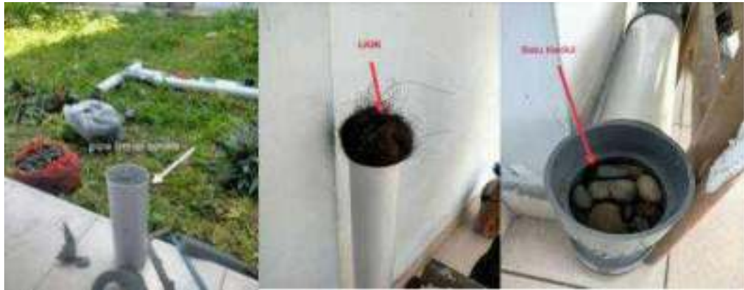
Gambar 4.2 Proses pengisian bahan material filter
