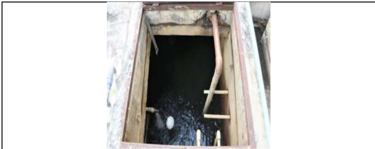
Use of Water Tanks Equipped with Balls (Automatic Buoys) at the USU School of Public Health
