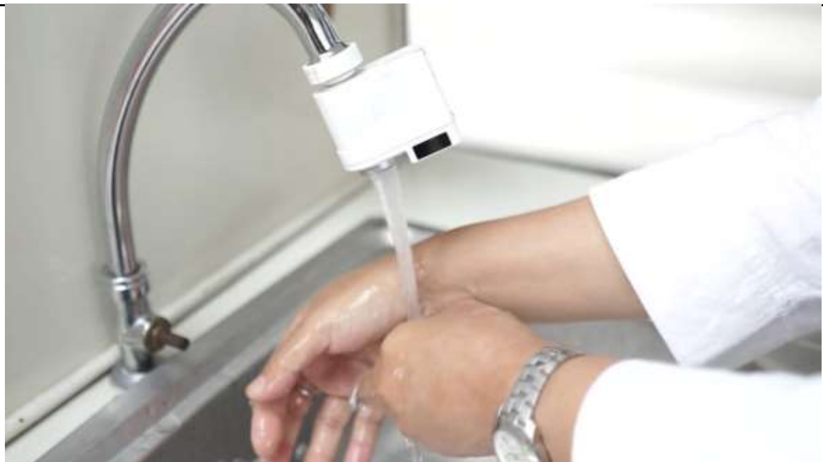
Sensor Water Faucet in Central Administration Building
