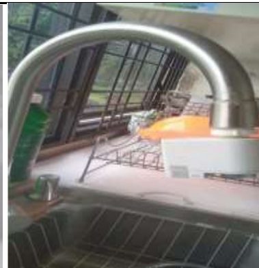
Use of water-saving faucets at the USU Integrated Research Laboratory and the USU Information Study Center
