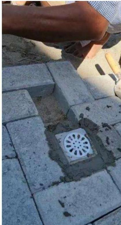
Penambahan lubang biopore diantara paving blok.
