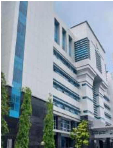
Gambar 13. Tampak Belakang Pembangunan Digital Learning Center Building
